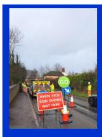
Operate units in line of sight of full set up at all times. End of shift, press button 2 for 2 sec to bring signs oblique (SiteSet Up mode). Turn off and remove.
